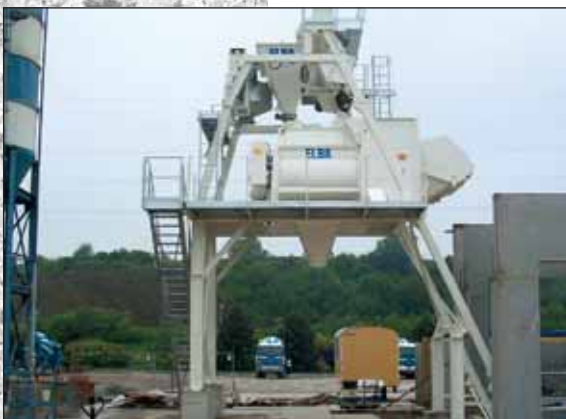
ELBA Beton-Center EBC D 130 während der Montage/ during erection
