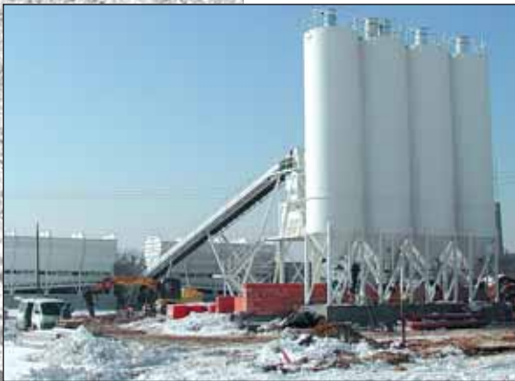
ELBA Beton-Center EBC B während der Montage/ during erection
